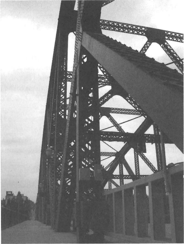
Broadway Bridge, Portland Jyndia Schaible © 2007
