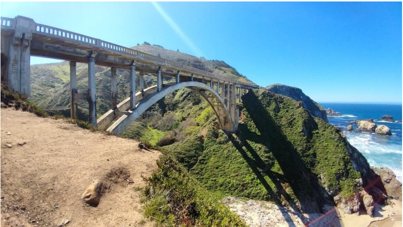
Rocky Creek Bridge © Garrett Broberg
